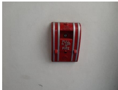
fire alarm manual station
